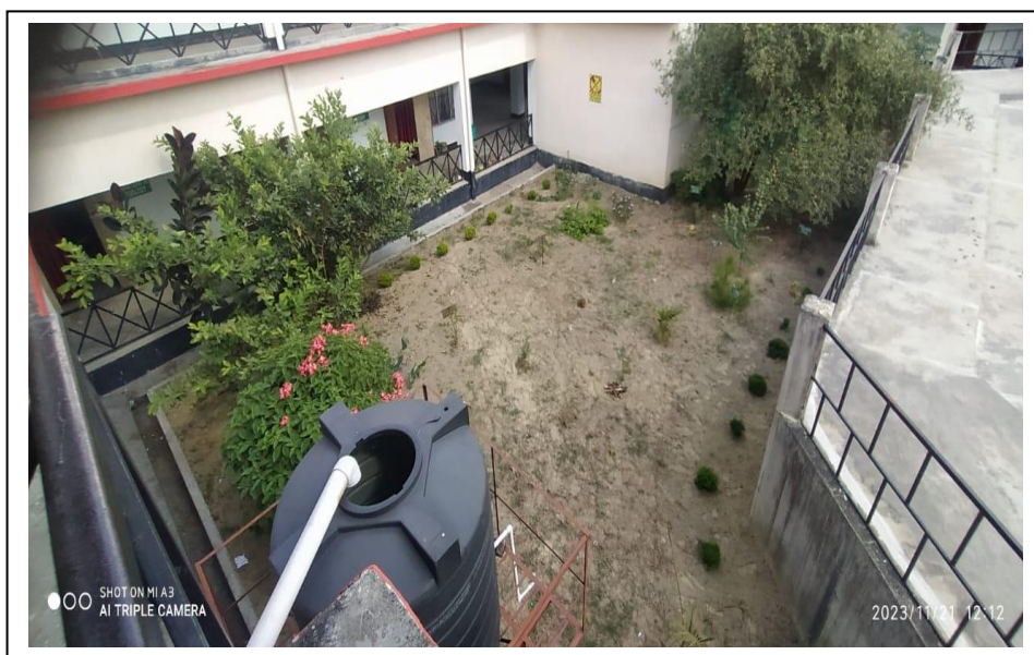
Photograph of tank showing collection of rainwater
